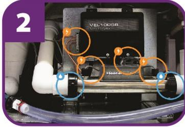
**2** Ensure all plumbing and electrical connections are securely connected and tightened as they can come loose during transit.
